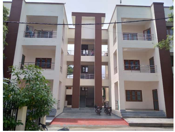
Residential Complex, Uttar Pradesh
